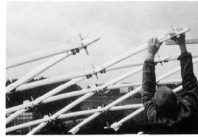
6.16 Assembly of the grid elements
