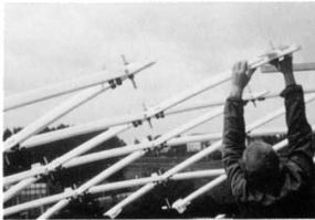
6.16 Assembly of the grid elements
